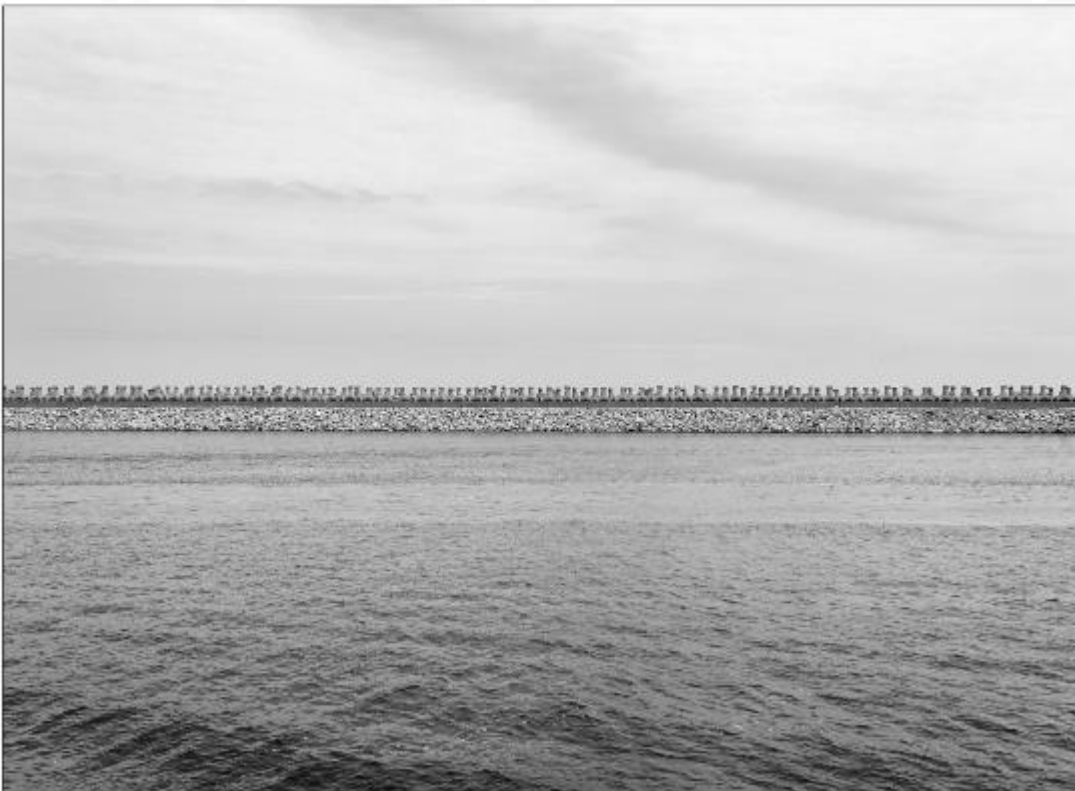
018 Breakwater Units - Leaving Constanta
