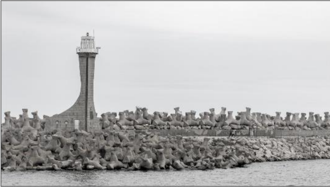
017 Breakwater Units - Leaving Constanta
